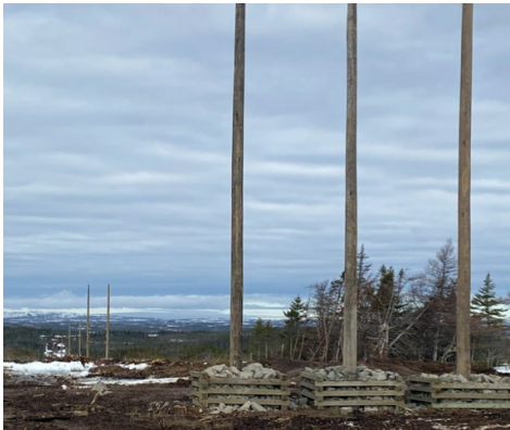
New H-Frame structures on transmission line 94L in the Blaketown area.
