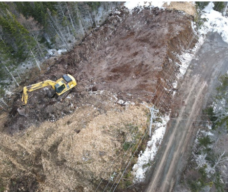
Vegetation work completed to improve access for Lockston substation project.
